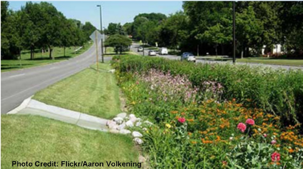
Example Bioretention Project
